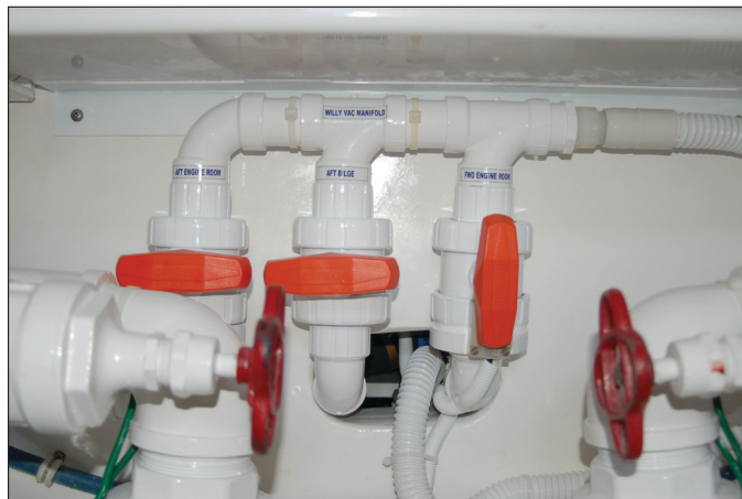
Figure 7: Manifold Assembly
