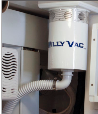
Figure 4: Vacuum Motor, Installed
